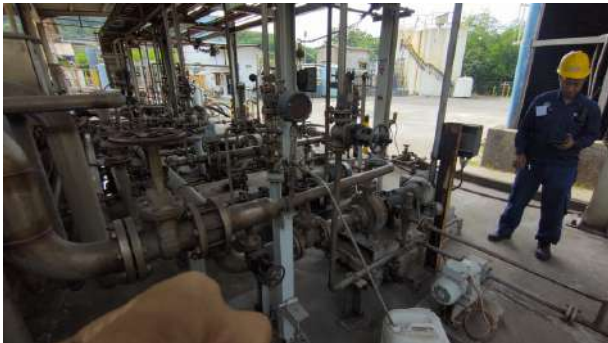
Gear Pump Maintenance at Indorama Polypet
