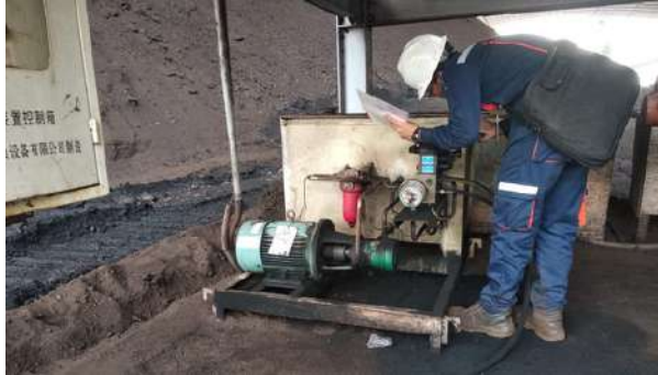
Hydraulic Power Unit Revitalization
